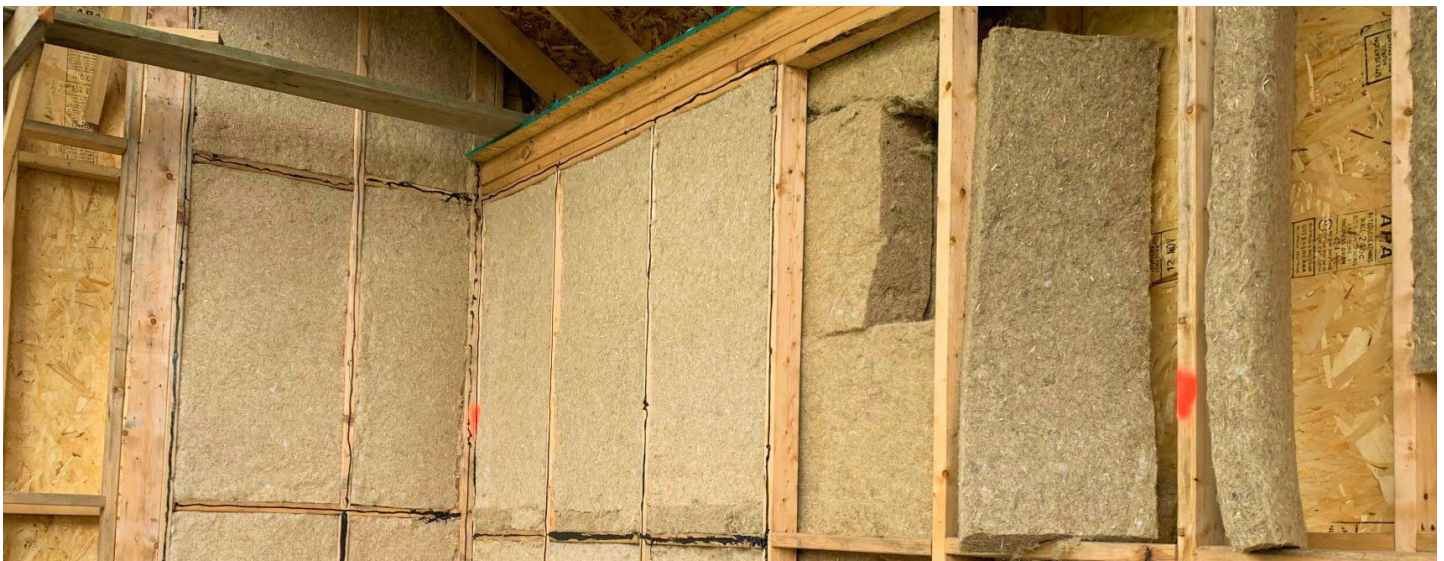
Photo 1. Installed Natur-Chanv/Hemp™ insulation panel
