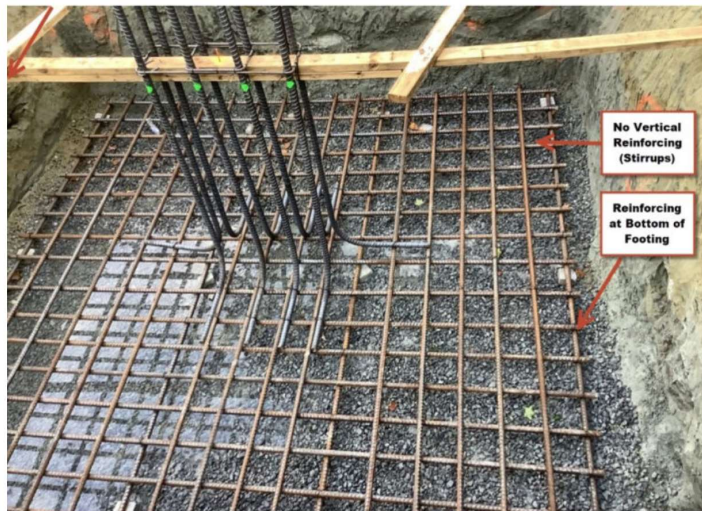
Figure 3 - Typical Pad Footing Construction
