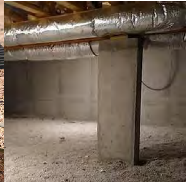
Crawlspace with Pad Footings
